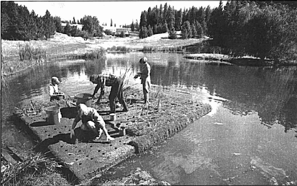
Karen Hayes, foreground, Todd Walker, left, Chris Hardy and Christy Latta work on top of a floating treatment wetland section being constructed for a pond near Hayden, Idaho. The Kootenai Environmental Alliance is preparing the experimental treatment wetland, to test the effectiveness in absorbing harmful nutrients in lakes and ponds.
